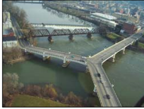
9 - The Y-bridge at Zanesville
