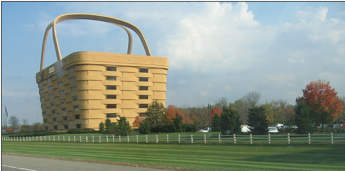
1 - The Headquarters of the Longaberger Basket Company at Newark, Ohio (from Route 16)
