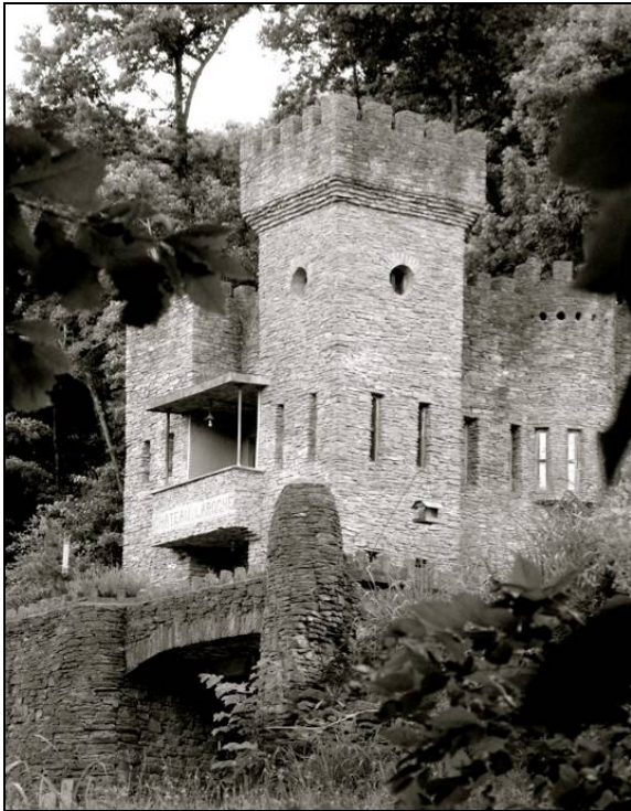
6 - Chateau La Roche at Loveland
