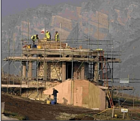
Work continuing on the Clavel Tower at Kimmeridge [2]
