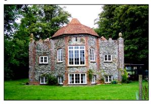
Hop Castle was left derelict for many years but has recently been renovated. This included the introduction of a new damp-proof course and underpinning of the foundations. All the windows were replaced and four additional windows added to the front elevation and a conservatory added to the side. As a result it has been returned to a two-bedroom private residence.
