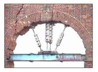
Park Newsletter (<u>www.brookmans.com</u>) has been reporting damage to the folly for some time, and the arch has had to be supported on a steel brace to stop it from collapsing.
