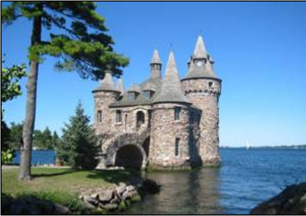
The Power House at Boldt Castle [1]
